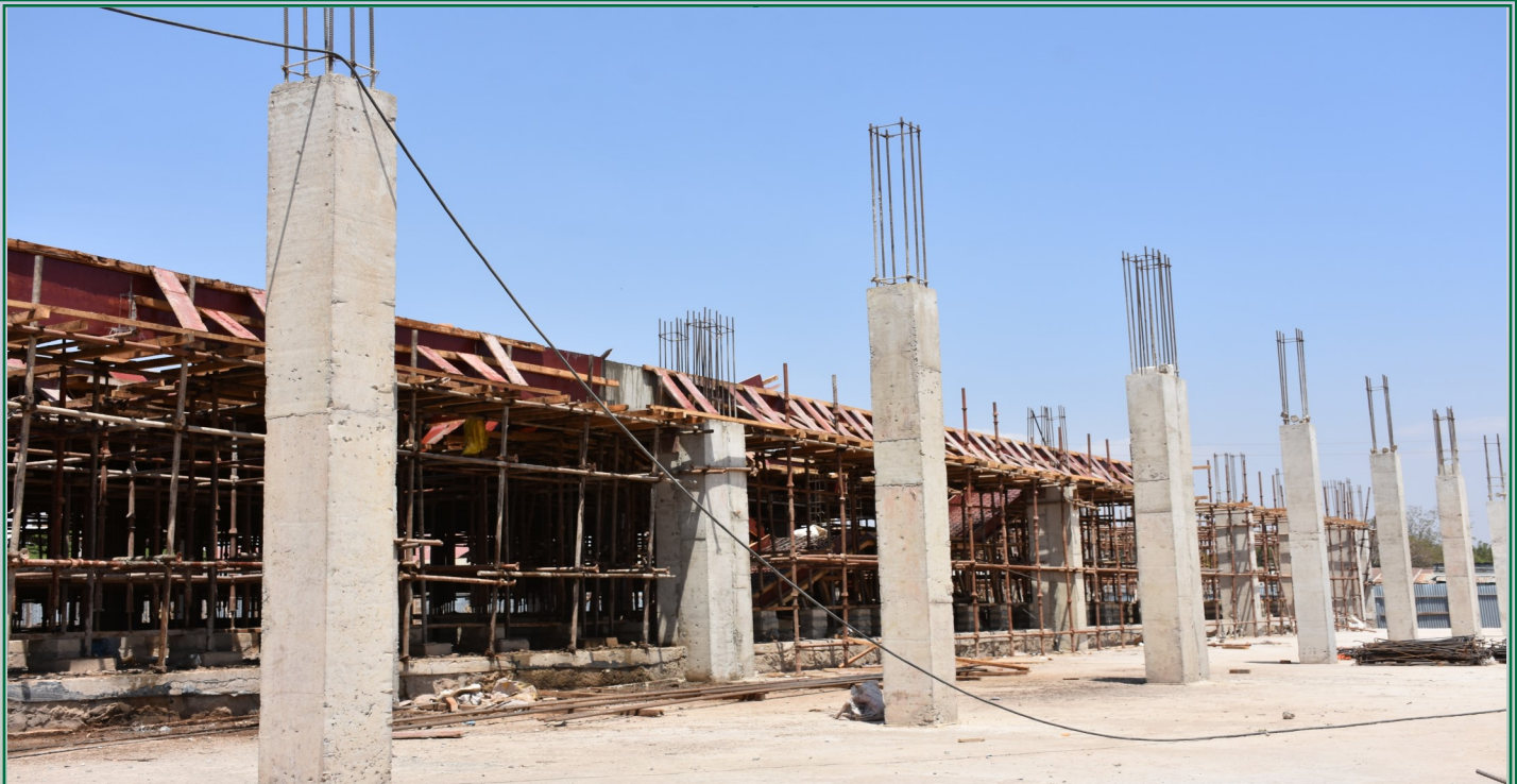
A section of Isiolo Modern Market under construction
