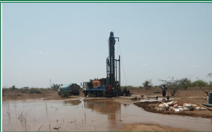
A borehole drilled by the County Government of Isiolo in Merti Sub County to reduce the shortage of water in the area.
