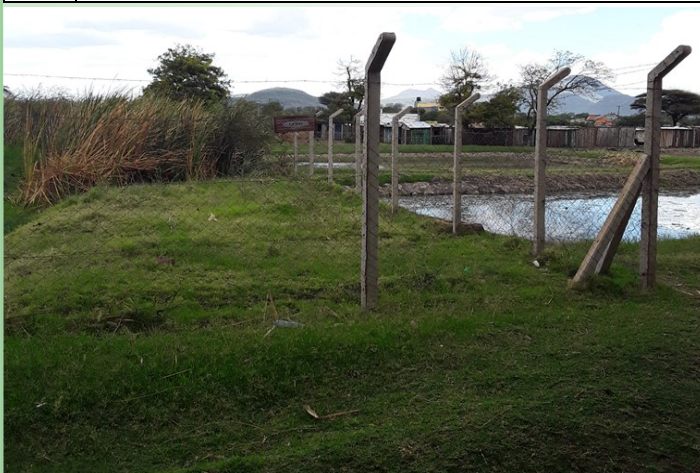
Fencing of concrete fish ponds and fish kiosk
