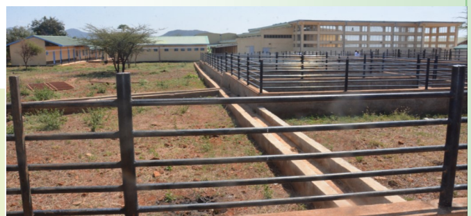
Camel Holding Segment and Bush Clearing done
