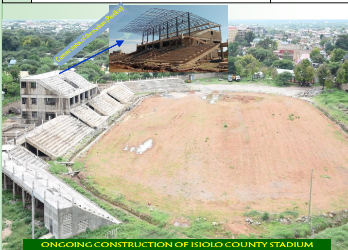
ONGOING CONSTRUCTION OF ISILOLO COUNTY STADIUM
