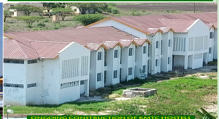
ONGOING CONSTRUCTION OF KMTC HOSTELS
