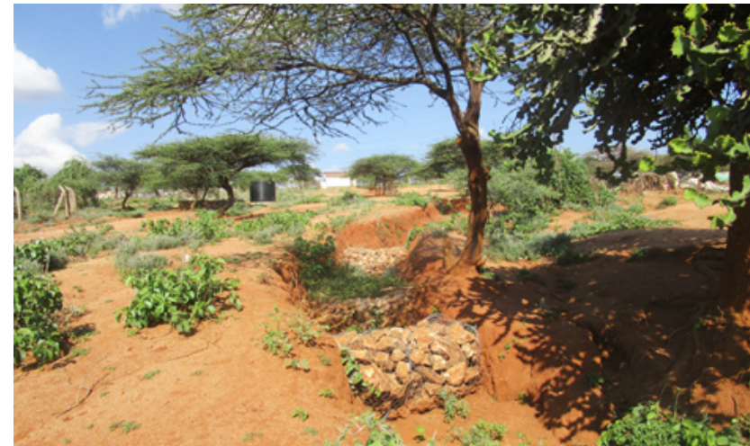
Plate 5.9: Control of soil erosion in Oldonyiro using gabions (Source: RCMRD)
